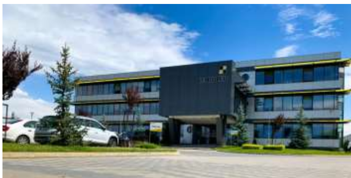
Electric Plus (Barrier)
